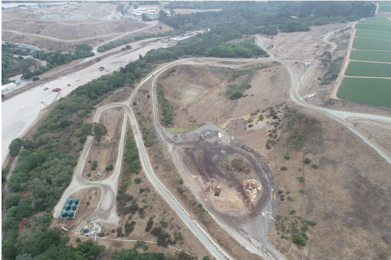
Aerial Photo of Landfill Phase IV
