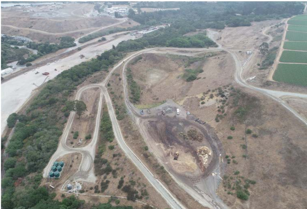
Aerial photo of Landfill Phase IV
